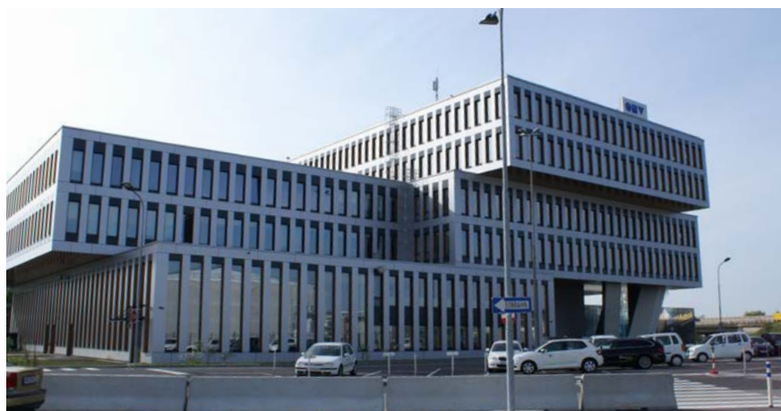
OMV Office Building, Mannswörther Straße 28, 2320 Schwechat Bitumenbahnen E-ALGV-4 | 3750 m 2 , E-KV-5 | 1 200 m 2
